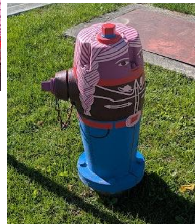
Fire hydrant in front of Trapnell
